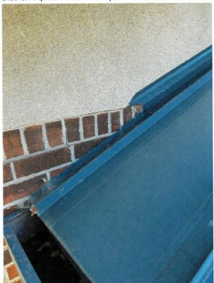
At another location the end wall flashing is not sealed correctly to the end wall. Again, the overhang has probably saved some problems. This should be sealed. It will require incorporating a kickout flashing as well and maybe a counter flashing. A counterflashing would go over the current flashing and be similar to the detail below.
