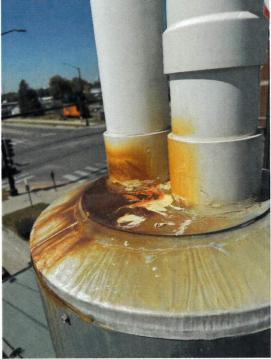
The flues are close to the next higher roof height and probably need to be as high as they are to exhaust properly. If they can be installed lower, a shorter base could replace the old flue and a univeral cap could be installed similar to photo below. Combined with the roof jack size there could be a way to remove some of the problem areas.
