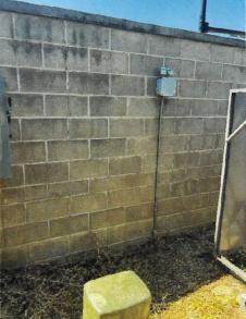
There are also areas where the brick itself is damaged or cracked. Most appears to be related to water freeze/ thaw damage. Faces of the brick have popped off and were laying on the ground next to the wall. Control joints weren't present and could be related to some cracking at the corners. It also might be possible that the wrong mortar was used in the brick (too hard or strong) and a softer mortar would potentially prevent some of the brick faces from popping off.
