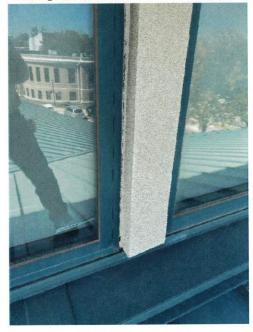
We also did a quick review of the masonry. The windowsills which we would call a sky facing joint should all be addressed. This also includes the tops of the screen walls. Some have been caulked. Properly done the caulking does a good job but they are still a maintenance issue and should be reviewed every year since they are all visible from the ground.
