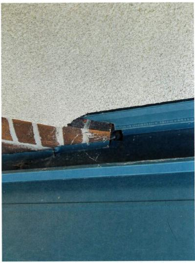
Another location has some water damage at the EFIS. There is no kickout flashing present. That type of flashing wasn't really a term when this was built but has become a code required item as a result of some poor installations. It's going to be a variation of the detail shown below but the end result is the same. This should be added at all locations where the eave does not extend past an adjoining wall.
